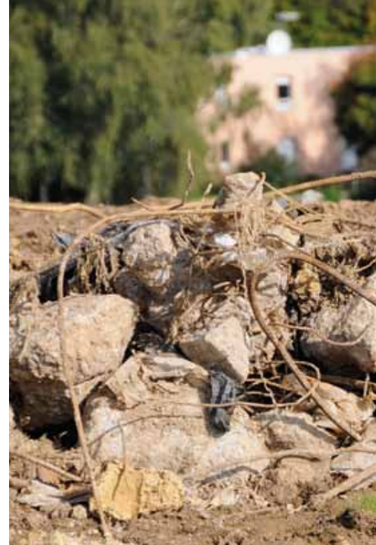
Entire blocks of flats have disappeared underground.
